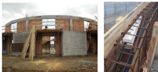
Figure 3.6. The ring beam reinforcement of the Church of St. Peter's and Paul's Bodzanow: (a) view of the completed reinforced concrete and (b) ring beam reinforcement (Szydłowski, 2017).
