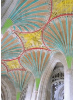
Figure 1.9. Fan vault components. Brown: masonry conoids; Red: horizontal circular rib on top of the conoids; Blue: congruent vertical ribs positioned at equal angles; Green: Tas-de-charge; Yellow: spandrel. Photo by Steve Cadman, Peterborough Cathedral, donated for free use, https://commons.wikimedia.org/wiki/File: Peterborough_retrochoir1.jpg , cropped and coloured by Bagi (2021).
