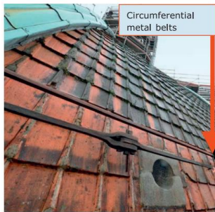
Figure 3.3. Metal bars on the Church of Umilta (Foraboschi, 2014).
