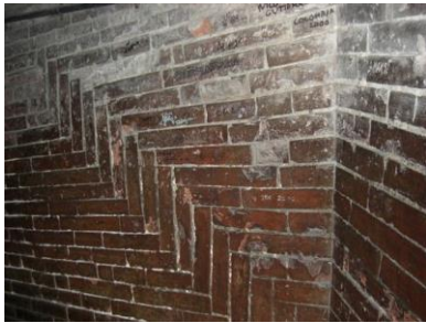
Figure 1.4. Herringbone patterns in Brunelleschi's dome.
