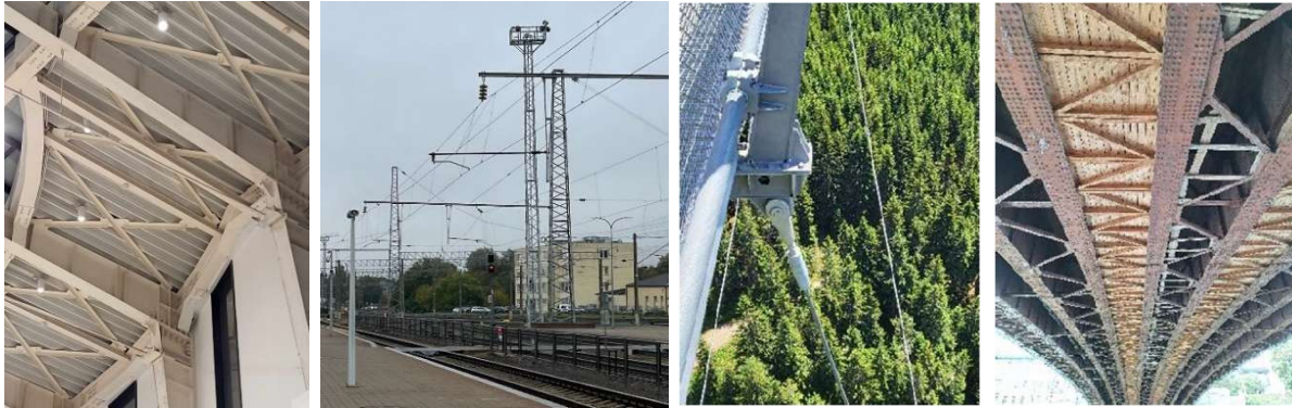
Figure 7: Pictures taken by students: roof structure of a shopping centre, railway transmission lines and a watchtower, cable connection detail, steel bridge underside
