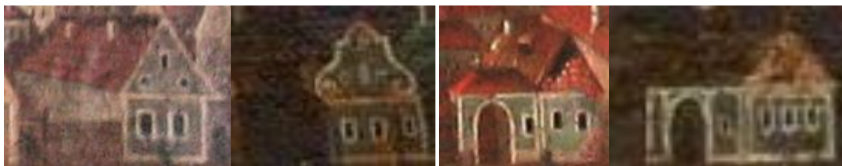
Fig. 5 – The house with displaced roof [8] (left) and overturned gables (right).
