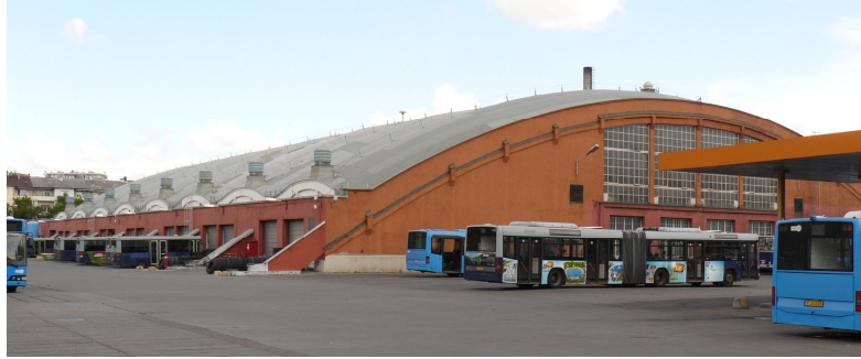
Figure 1.2.: Reinforced concrete shell structure of Kelenföld bus garage, Budapest (photo by the author)
