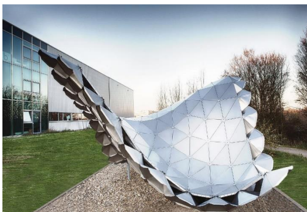
Fig. 1. Prototype 1 based on faceted plane components.
