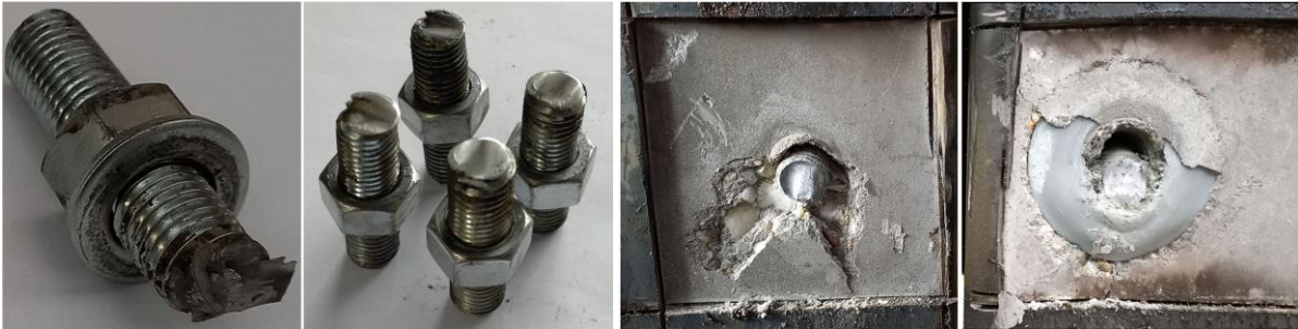
Figure 6. Failure of the bolts (left), concrete cracking and mortar filling with bolt deformation (right)
