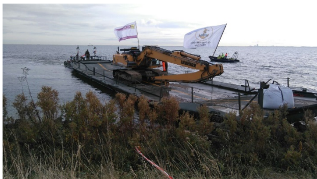
Figure 7. Exercise Waterwolf, Marken, The Netherlands, 2-4 November 2016: placing of Big Bags by the military.
