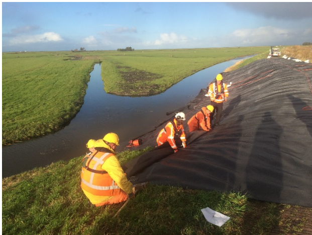
Figure 1. Erosion protection measure (inner slope).
