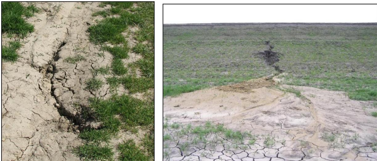
**Fig. 1.** Typical surface cracking on an embankment crest (Cibakháza, 2013), washed-out dispersive clay from an embankment (Tiszabura, 2012)
