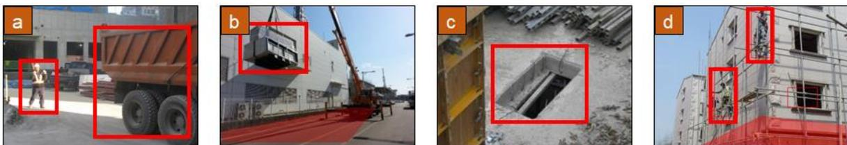
Figure 16 Determination of risk zones:(a) worker entering to the proximity zone (b) risk zone under lifted material by crane (c) controlled zone around the opening in floor (d) controlled zone for the scaffolding work.
