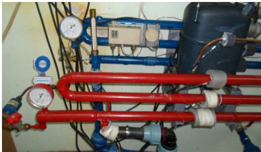
**Figure 2.4.** Mass flow measurements
